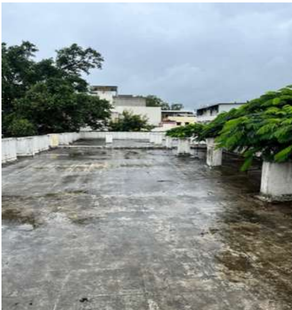
Figure 16 School 27 and 28 : Terrace (2)
