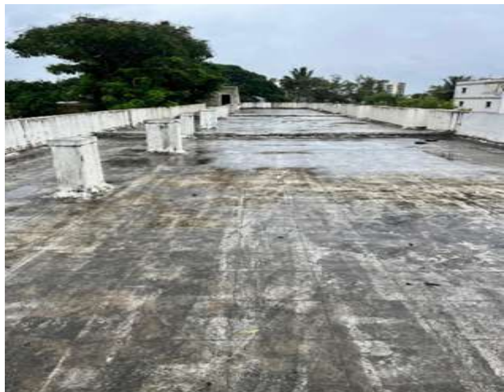
Figure 15 School 27 and 28 : Terrace (1)
