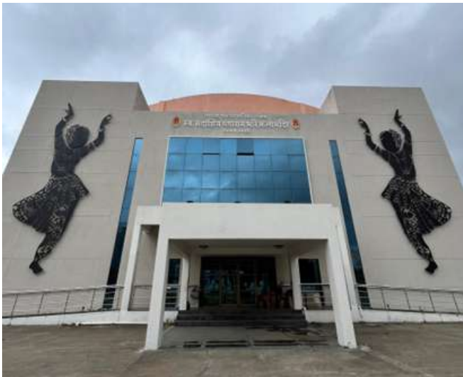
Figure 21 Sadubhau Bhore Natyagrug : West Facade
