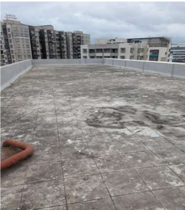
Figure 26 Atal Divyang Bhavan - Terrace (1)
