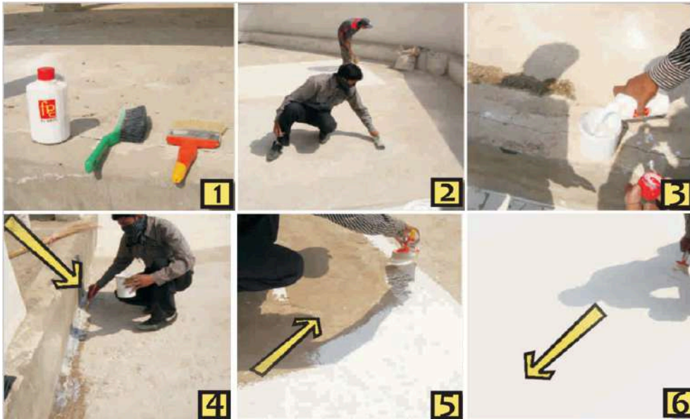
Figure 6 Step by step process for the application of cool roof paint
