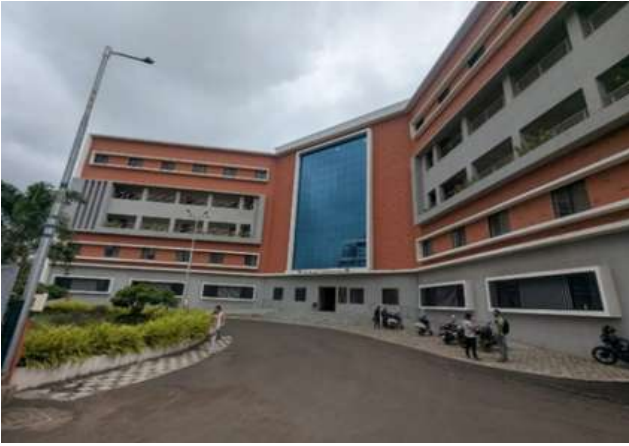
Figure 24 Atal Divyang Bhavan - Entrance
