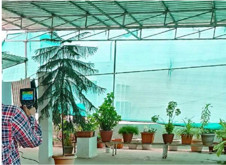
Figure 9 Walkthrough survey observation of rooftop green net shading, a widely adopted household measure for reducing indoor heat in Amravati
