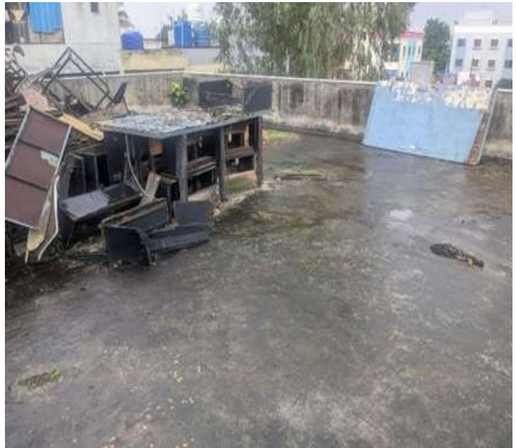
Figure 17 School 27 and 28 : Terrace (3)
