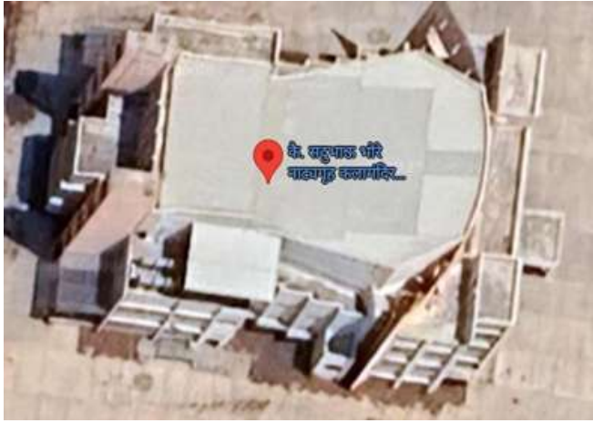
Figure 19 Sadubhau Bhore Natyagrug : Roof view
