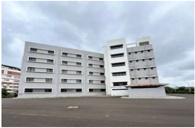
Figure 25 Atal Divyang Bhavan - East Facade
